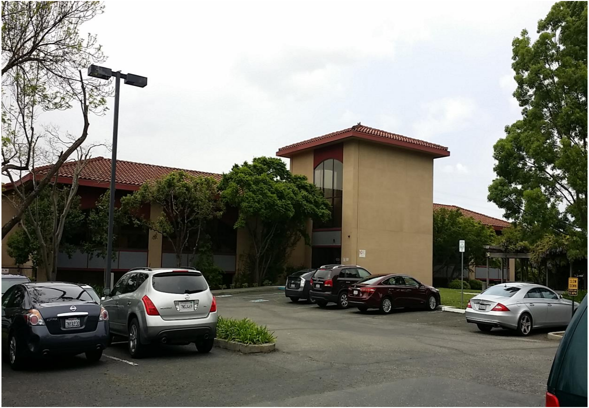
2 Subject Site Backside.
