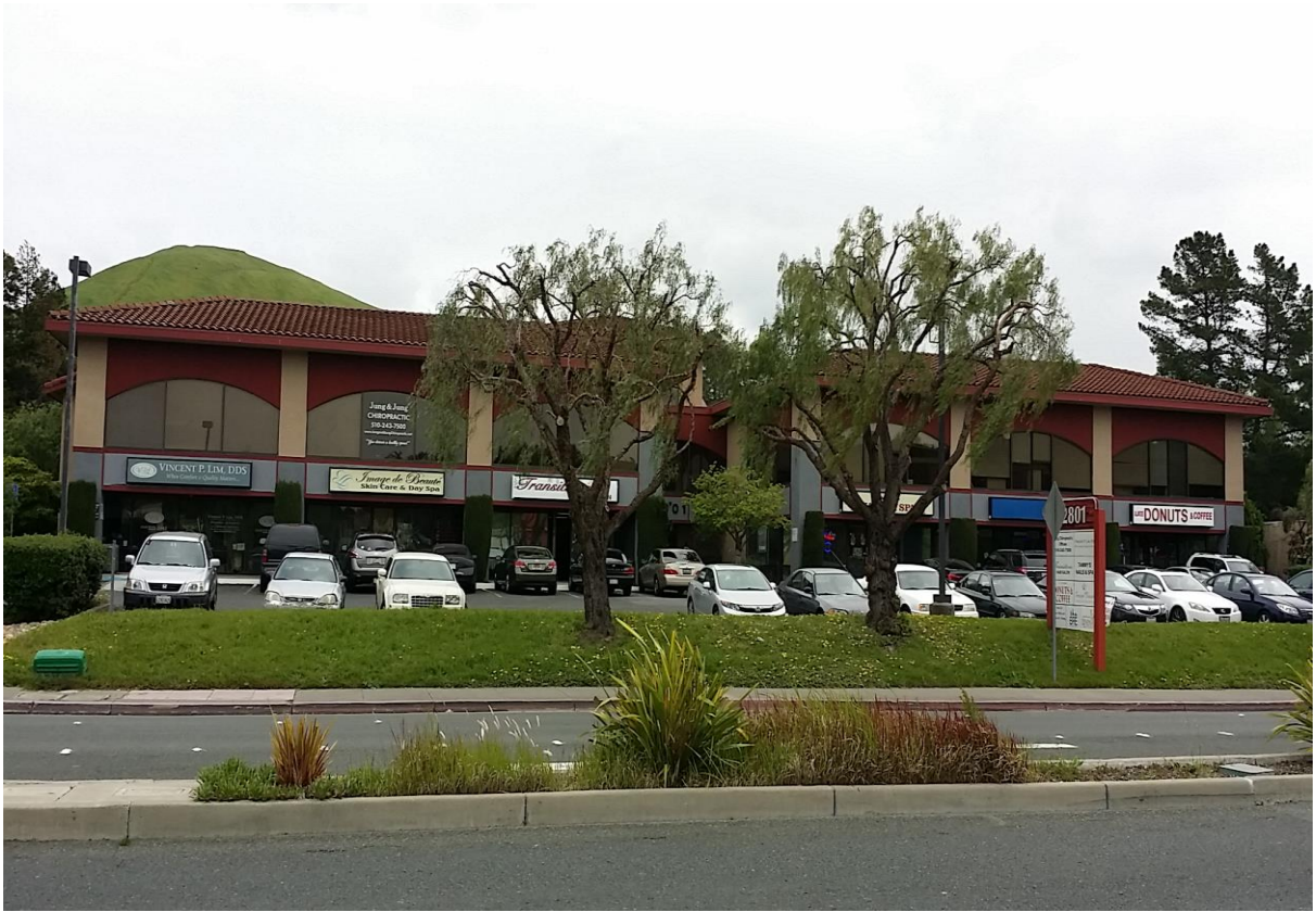
1 Subject Site Front side viewed from across Pinole Valley Road.
