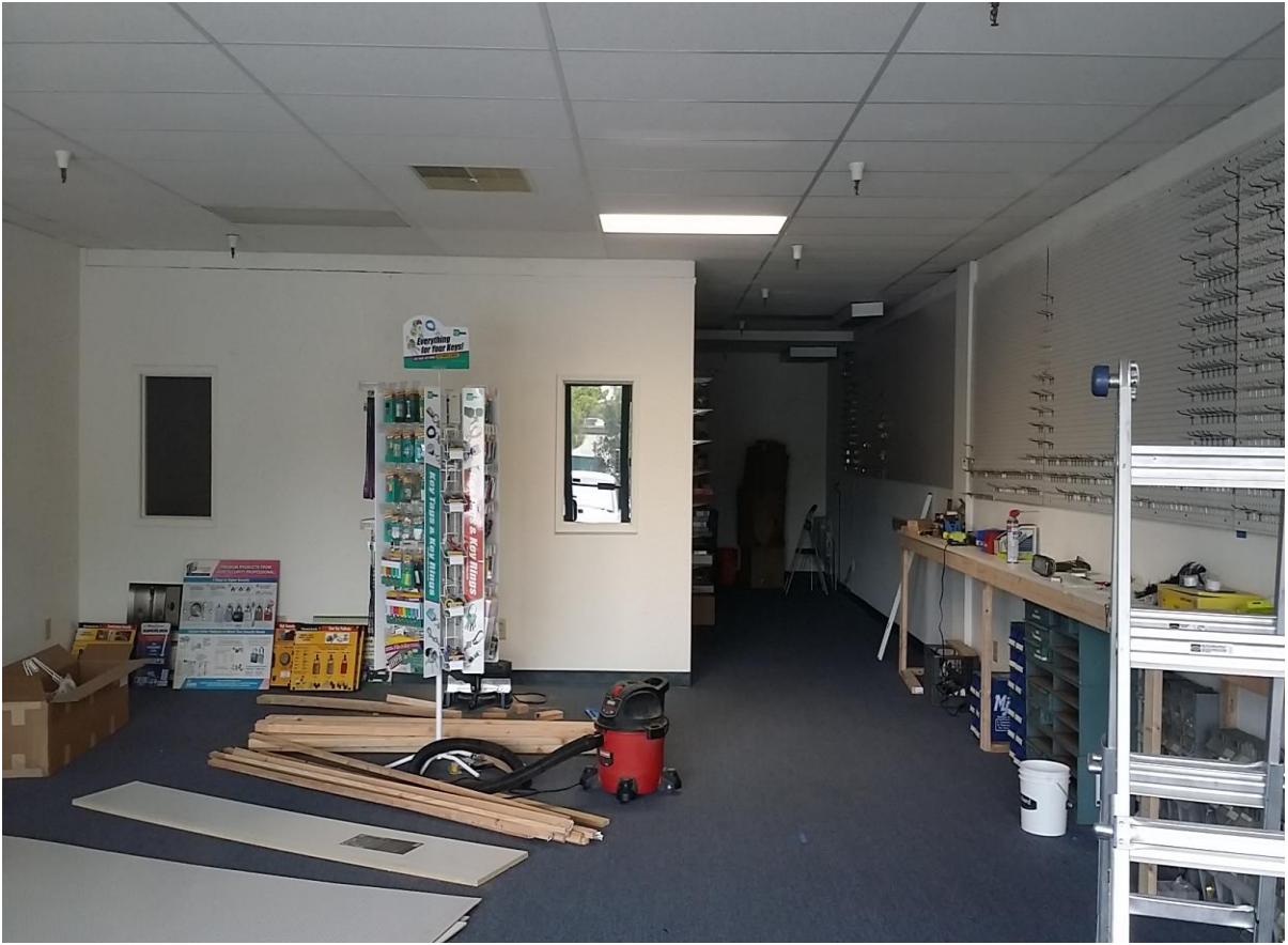
5 Subject Site Armor Locksmith undergoing tenant improvements.
